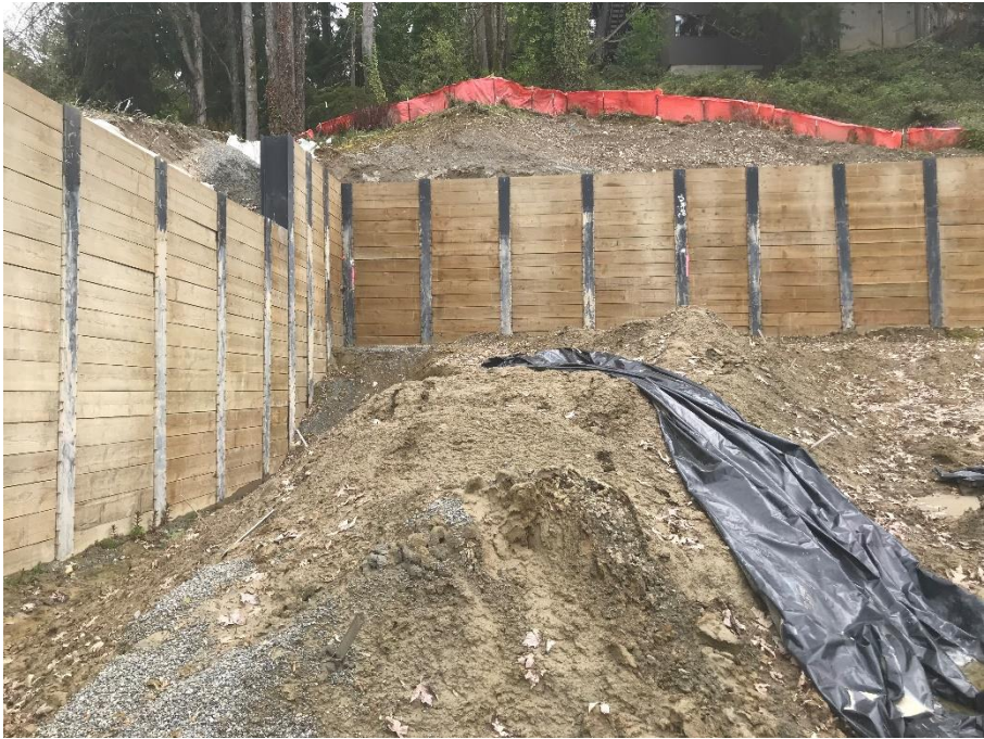
Photograph 2. North and east shoring walls
