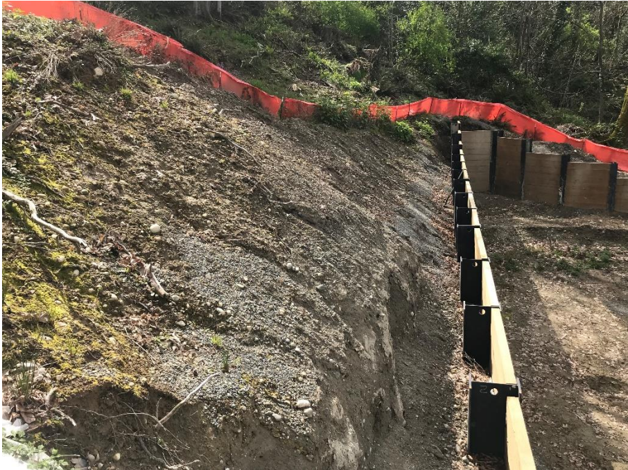
Photograph 5. Cut slope above east shoring wall, looking south.
