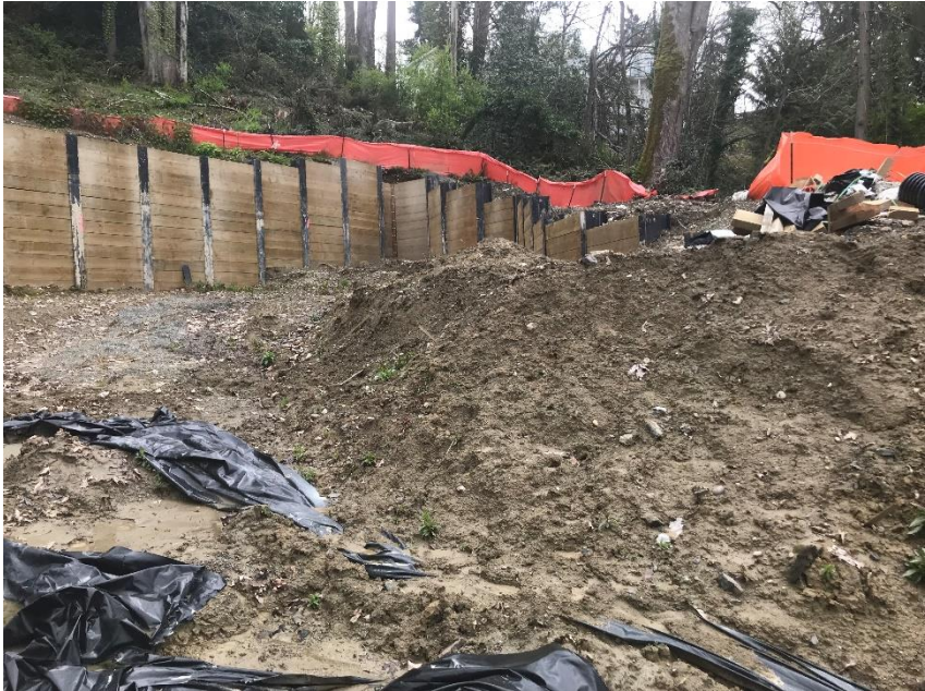
Photograph 3. East and south shoring walls
